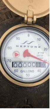
You should read the meter like a car odometer. You should read the meter from left to right and include the last zero on the meter. If the small black/red triangle or star (leak detector) is moving, water is going through your meter. This means that you have something on or you have a leak.
